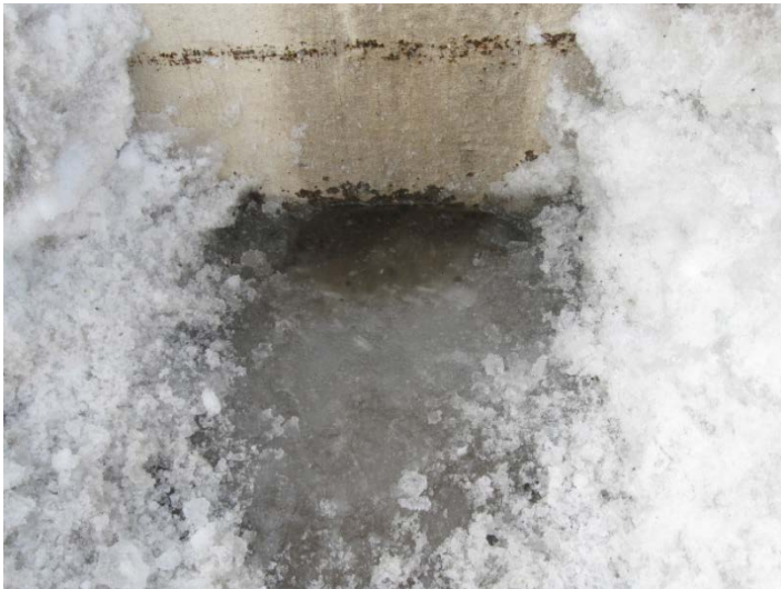
Photo 015: South railing base
