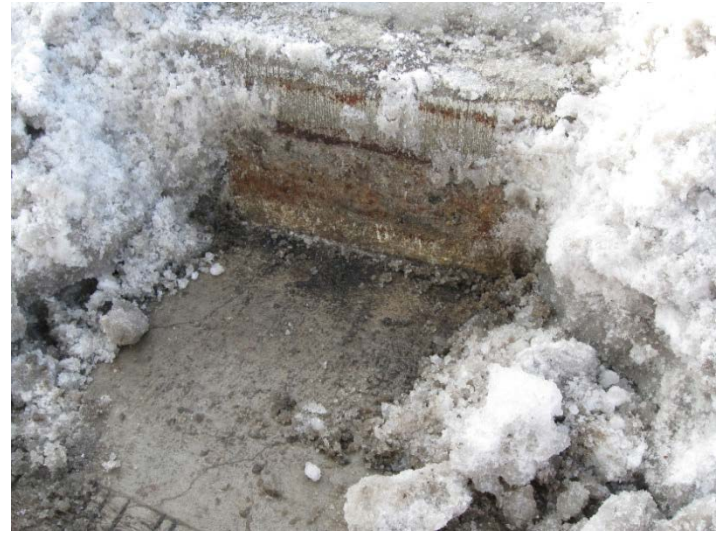
Photo 014: South curb line
