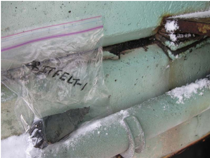
Photo 007: Bituminous felt sample
