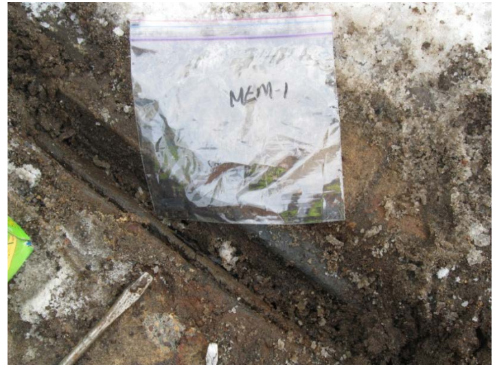
Photo 012: Expansion joint membrane
