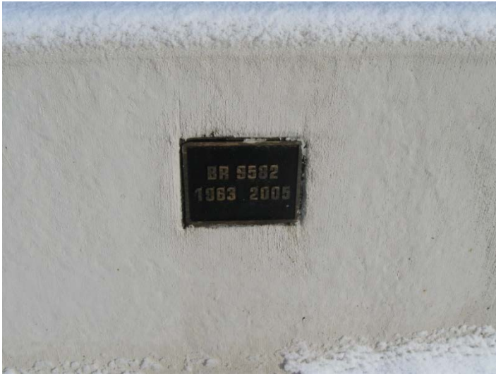
Photo 001: Bridge 9582 Name Plate
