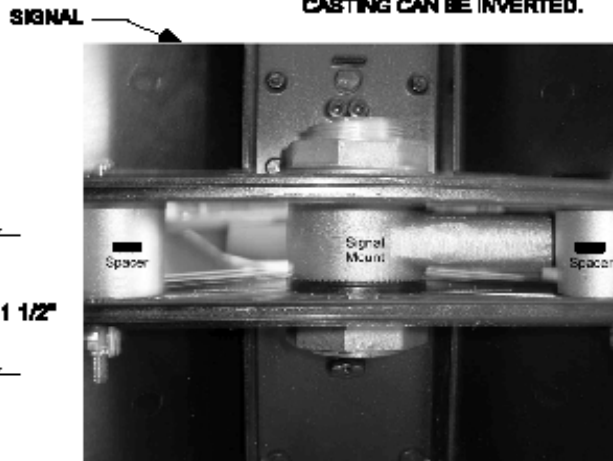
SHM Spacer Installed
