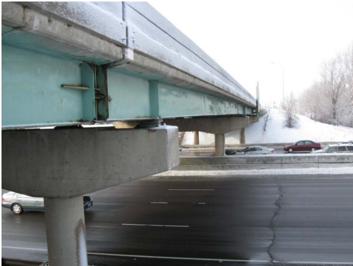
Photo 003: Supports from East
