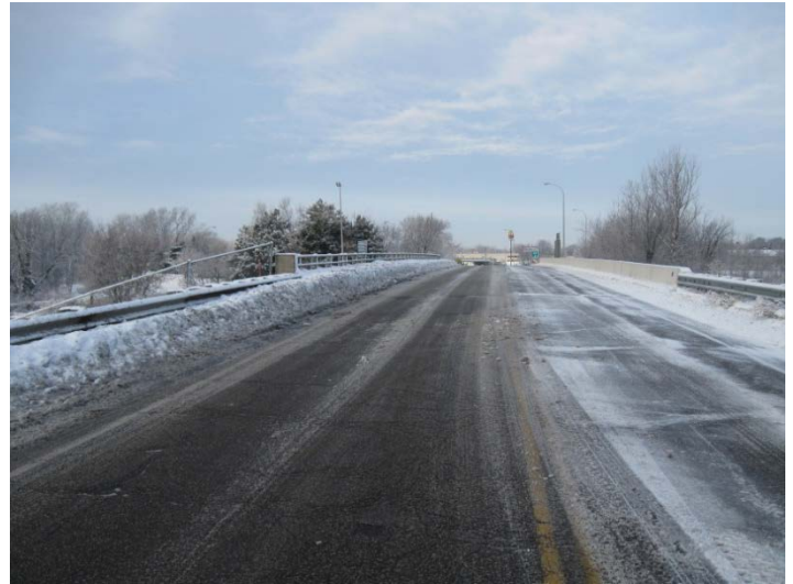
Photo 002: Bridge from East
