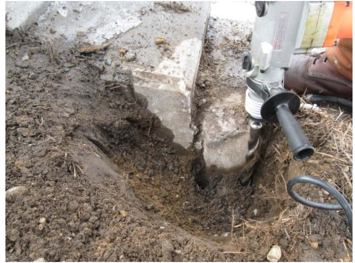
Photo 010: Probing for water proofing
