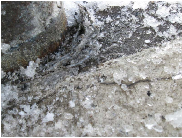
Photo 013: Lead shim under railing
