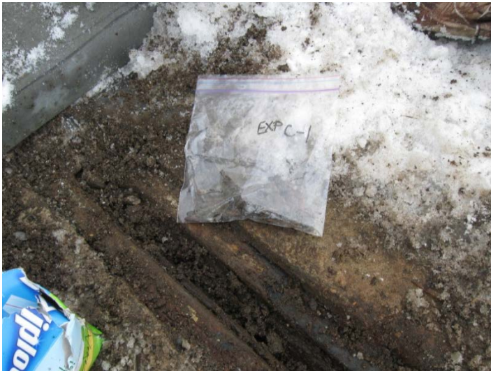
Photo 011: Deck Expansion Joint
