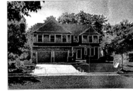
866 MONTANA AVENUE WEST (FRONT) SAINT PAUL, MINNESOTA
