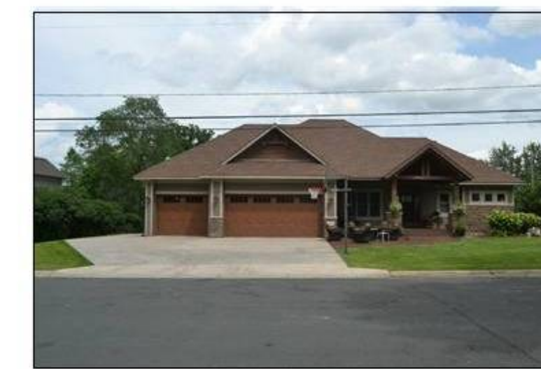
FRONT OF 3420 FAIRVIEW AVENUE NORTH CITY OF ARDEN HILLS, RAMSEY COUNTY, MINNESOTA
