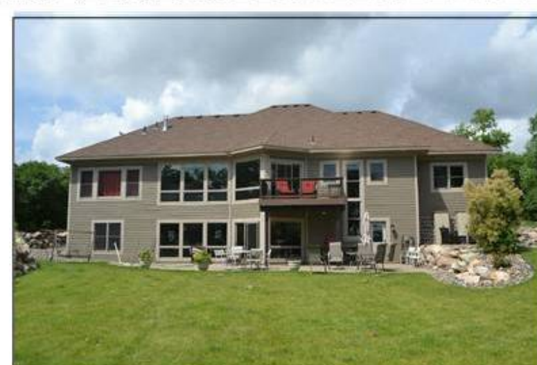
REAR OF 3420 FAIRVIEW AVENUE NORTH CITY OF ARDEN HILLS, RAMSEY COUNTY, MINNESOTA
