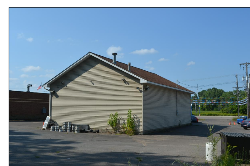
REAR OF 336 LARPENTEUR AVENUE WEST CITY OF ST. PAUL, RAMSEY COUNTY, MINNESOTA
