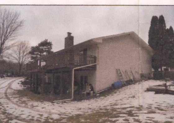
NORTHEASTERLY SIDE OF 1779 LAKE VALENTINE ROAD CITY OF ARDEN HILLS, RAMSEY COUNTY, MINNESOTA
