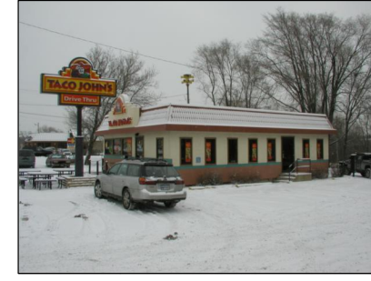
ADJACENT "TACO JOHN'S" (NOTE THAT PARKING LOT AND STEPS ENCRIDGE ONTO SUBJECT PROPERTY)
