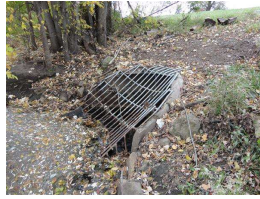
3. bridge safety 043.JPG
