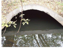
2. bridge safety 042.JPG
