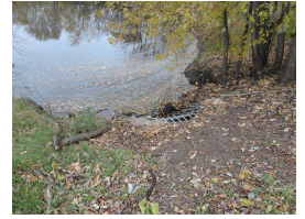
5. bridge safety 045.JPG
