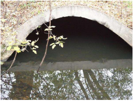
1. bridge safety 041.JPG
