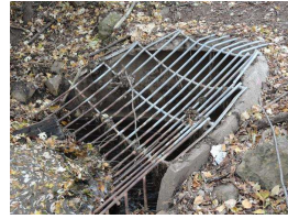
4. bridge safety 044.JPG
