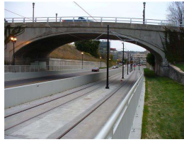
23. elevation view east_2_10-29-2013.JPG
