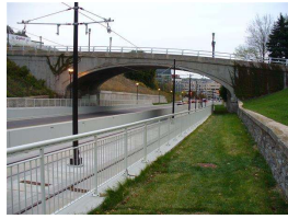
22. elevation view east_1_10-29-2013.JPG
