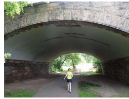
13. side view facing E.JPG
