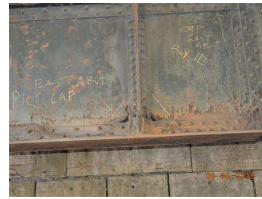
19. pier cap - E.side N.inside bay_1zoomWest.JPG
