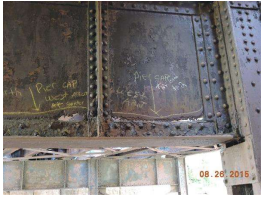
36. pier cap - W.side N.inside bay_1zoomWest2.JPG
