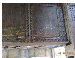
33. pier cap - W.side N.inside bay_1zoomWest2.JPG
