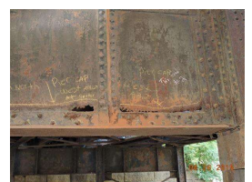
35. pier cap - W.side N.inside bay_1zoomWest1.JPG
