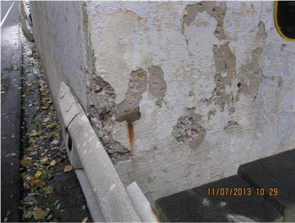
Photo 5 - SW corner of East pier wall 2013
