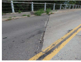
12. S Approach, SB lane.JPG
