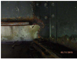
16. steel beam and bearing.JPG
