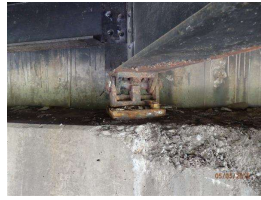
7. bearing N.abut - 3 beamline_1.JPG
