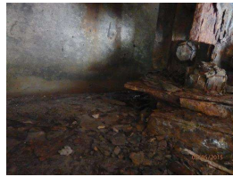
17. steel beam and bearing - SE corner.JPG
