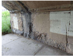
13. Abutment at sidewalk W side (4).JPG
