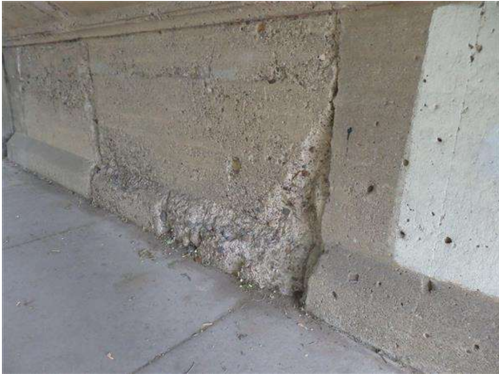
Photo 10 - Abutment at sidewalk W side (1)
