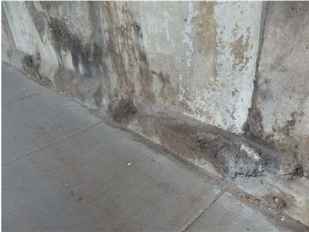
Photo 8 - Abutment at sidewalk E side (2)
