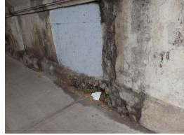
7. Abutment at sidewalk E side (1).JPG
