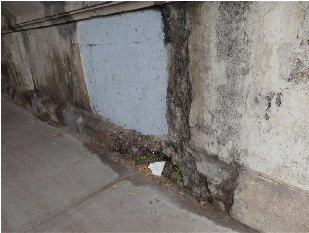
Photo 7 - Abutment at sidewalk E side (1)
