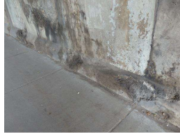
8. Abutment at sidewalk E side (2).JPG
