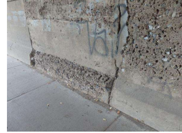
9. Abutment at sidewalk E side (3).JPG
