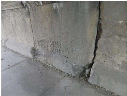
11. Abutment at sidewalk W side (2).JPG
