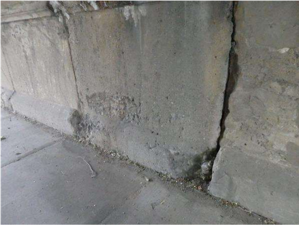
Photo 11 - Abutment at sidewalk W side (2)
