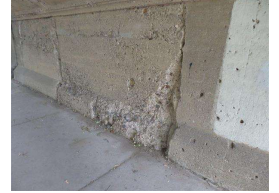
10. Abutment at sidewalk W side (1).JPG
