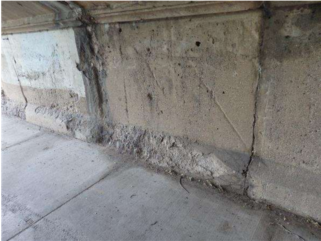
Photo 12 - Abutment at sidewalk W side (3)
