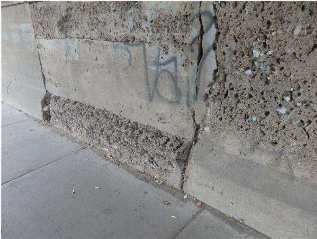
Photo 9 - Abutment at sidewalk E side (3)
