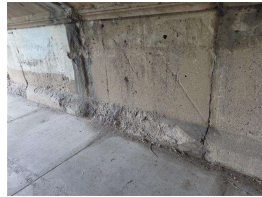
12. Abutment at sidewalk W side (3).JPG
