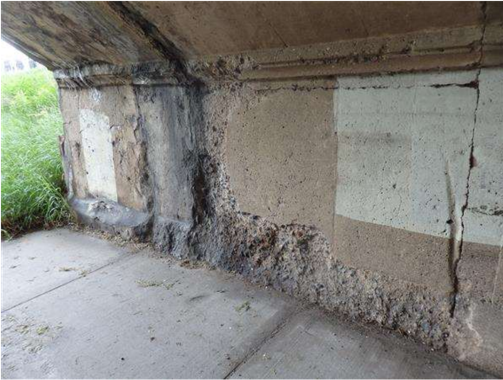
Photo 13 - Abutment at sidewalk W side (4)
