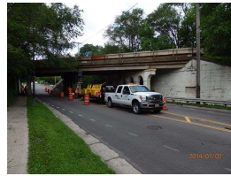
18. 035 abut and column repairs by - RR.JPG
