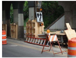
17. 034 abut and column repairs by - RR.JPG
