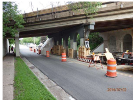
16. 033 abut and column repairs by - RR.JPG
