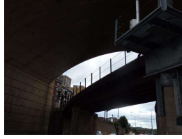
7. Metal rail, W side.JPG
