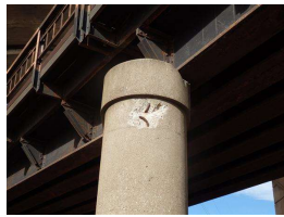
2. E end of center Pier wall.JPG
