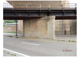
25. pier wall facing north.JPG
