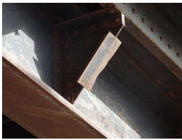
1. Cantilever brace over WB lane.JPG
