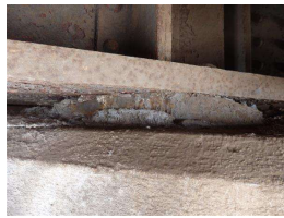
3. Fixed bearing, center Pier wall.JPG
