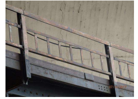
20. metal ped railing topside.JPG
