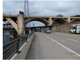
19. facing west view.JPG
