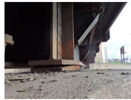
4. Fixed bearing, E side of center Pier wall.JPG
