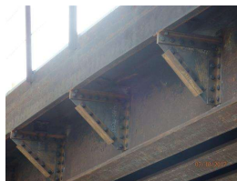
28. three cantilevers repaired 2016.JPG
