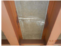
8. underdeck efflorescence_1.jpg
