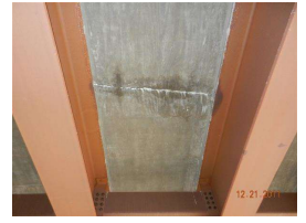
10. underdeck efflorescence_3.jpg
