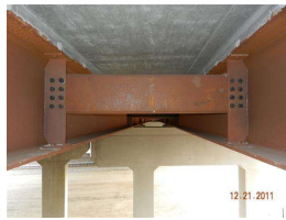
3. beams and diaphragm weathering steel.jpg
