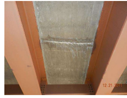
9. underdeck efflorescence_2.jpg
