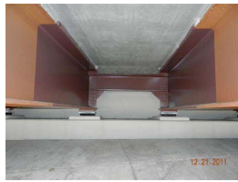
2. beam ends and diaphragm painted_2.jpg
