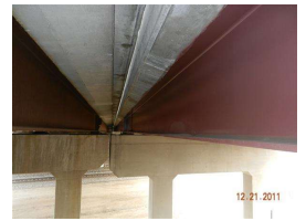
5. fascia beam painted.jpg
