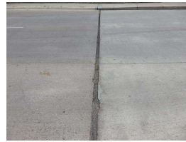
19. Approach relief joint at W end.JPG
