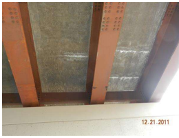
11. underdeck efflorescence_5.jpg
