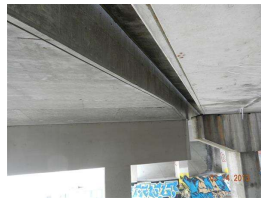
87. median joint East 029.jpg
