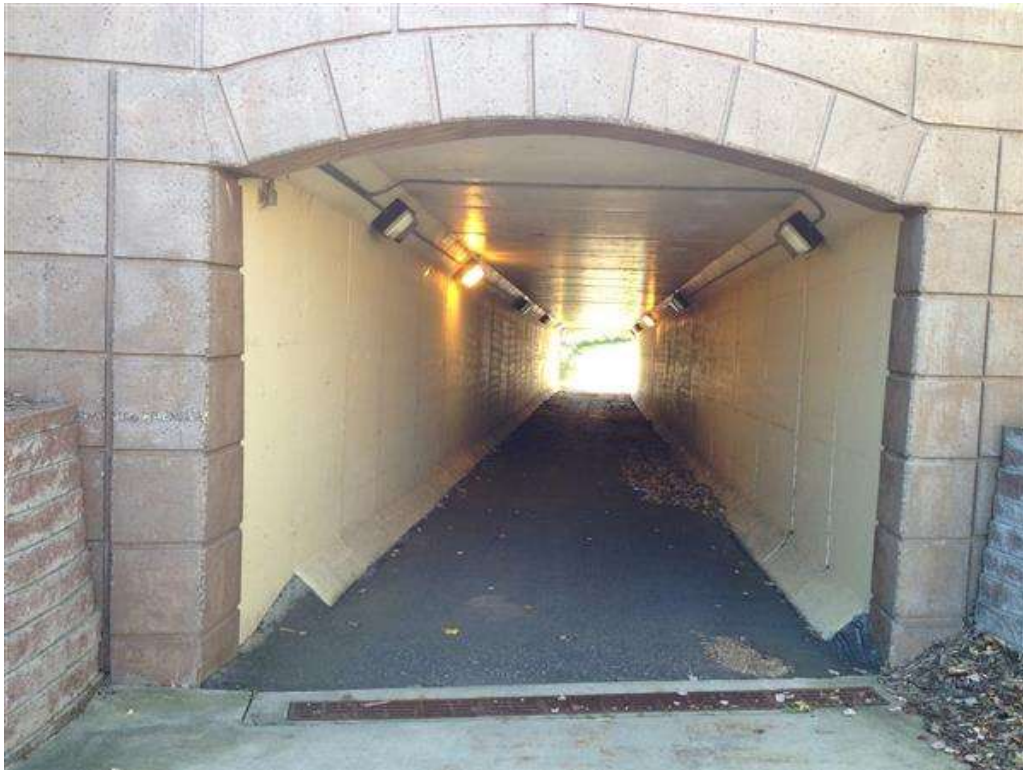
Photo 4 - Culvert Looking South
