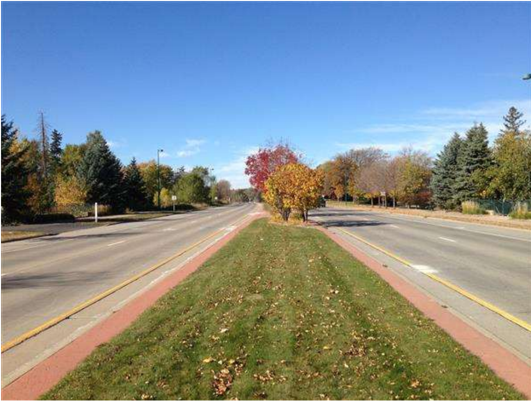
Photo 3 - Alignment View Looking West
