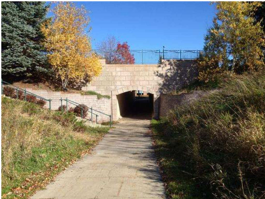
Photo 2 - Elevation View Looking North
