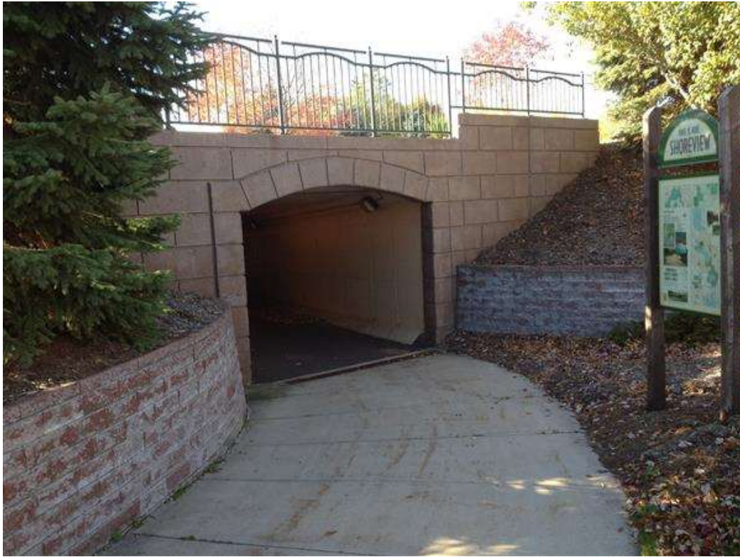
Photo 1 - Elevation View Looking SW
