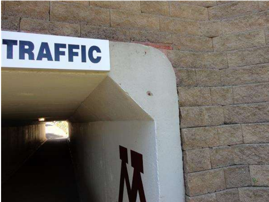
Photo 4 - SpallInNorthEndTunnel
