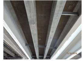
15. Between 1st & 2nd Pier Walls from the N.JPG
