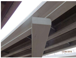
1. 1st Pier Cap, S end of bridge, W side (1).JPG
