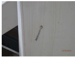
2. 1st Pier Cap, S end of Bridge, W side (2).JPG
