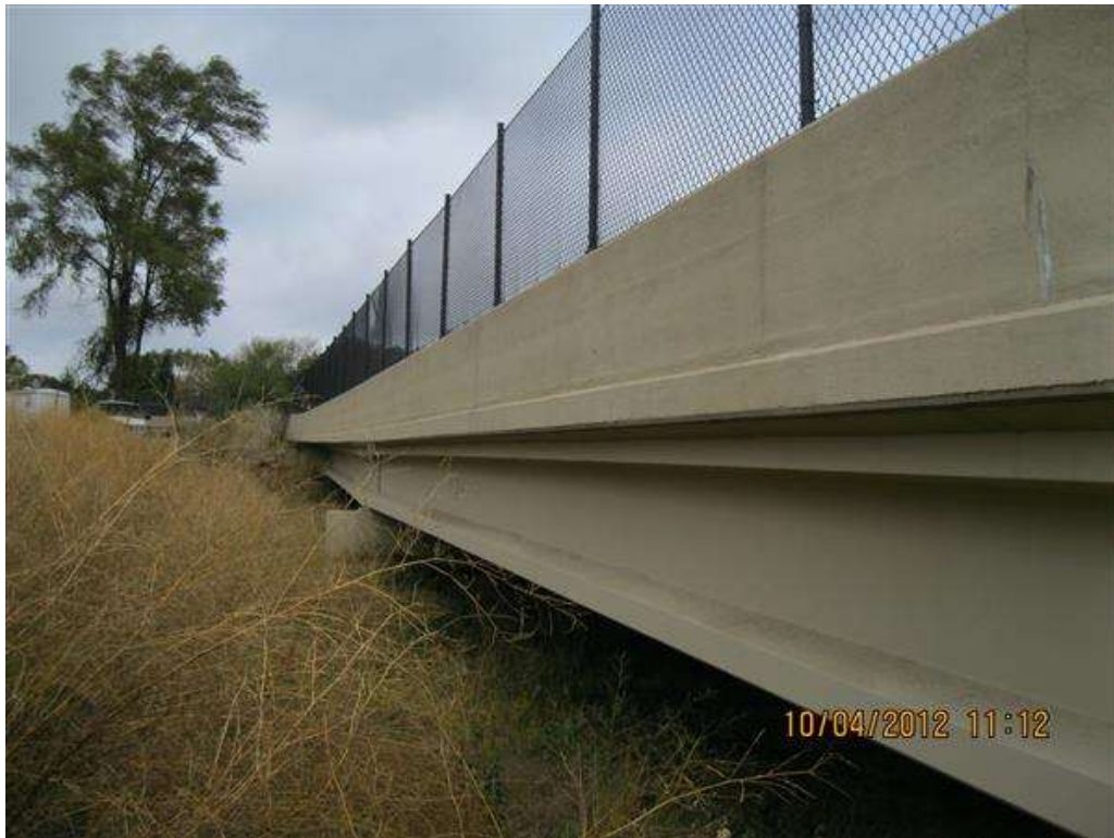
Photo 16 - West Bridge Rail
