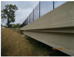
16. West Bridge Rail.JPG
