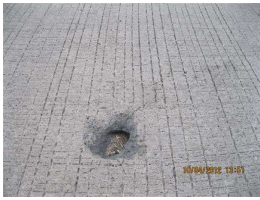
11. Overlay South side Pier #1 WB.JPG
