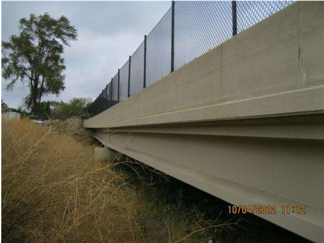
Photo 15 - West Bridge Rail
