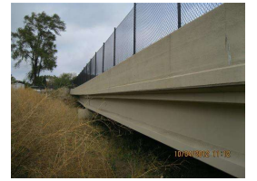
15. West Bridge Rail.JPG
