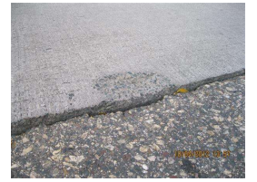
10. SW Corner South Approach Slab.JPG
