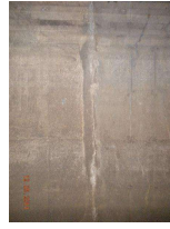
8. construction joint_1-4.jpg
