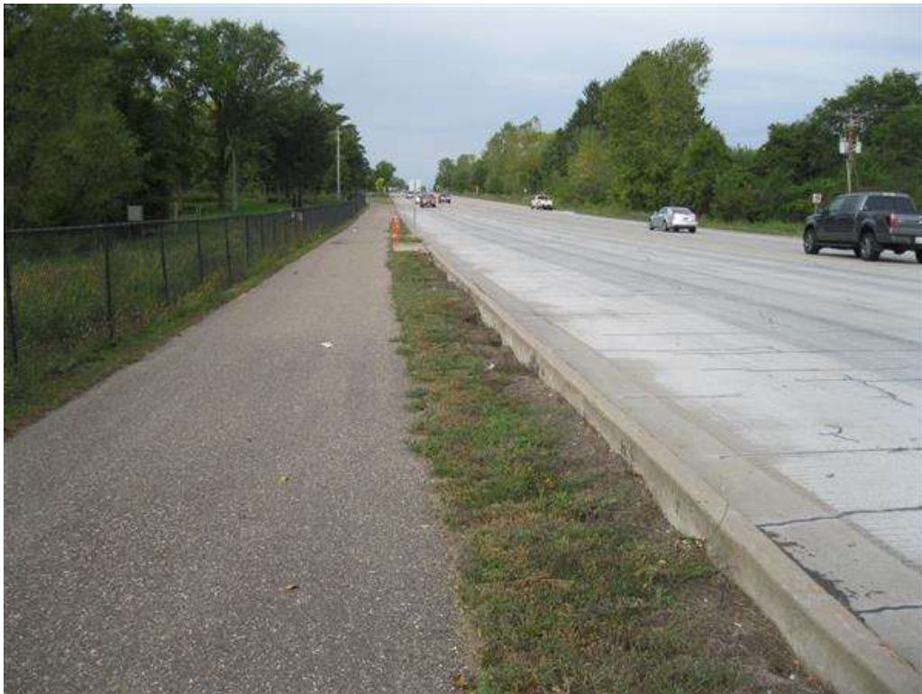
Photo 4 - curb south side.JPG
