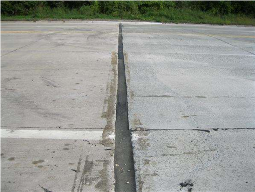
Photo 11 - west E-8 joint.JPG
