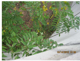
2. erosion @ NW wingwall-2.JPG
