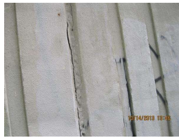
3. joint in SW wing wall.JPG
