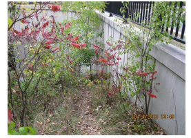
10. NW wing wall.JPG
