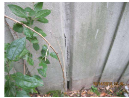
4. joint in SW wing wall-2.JPG
