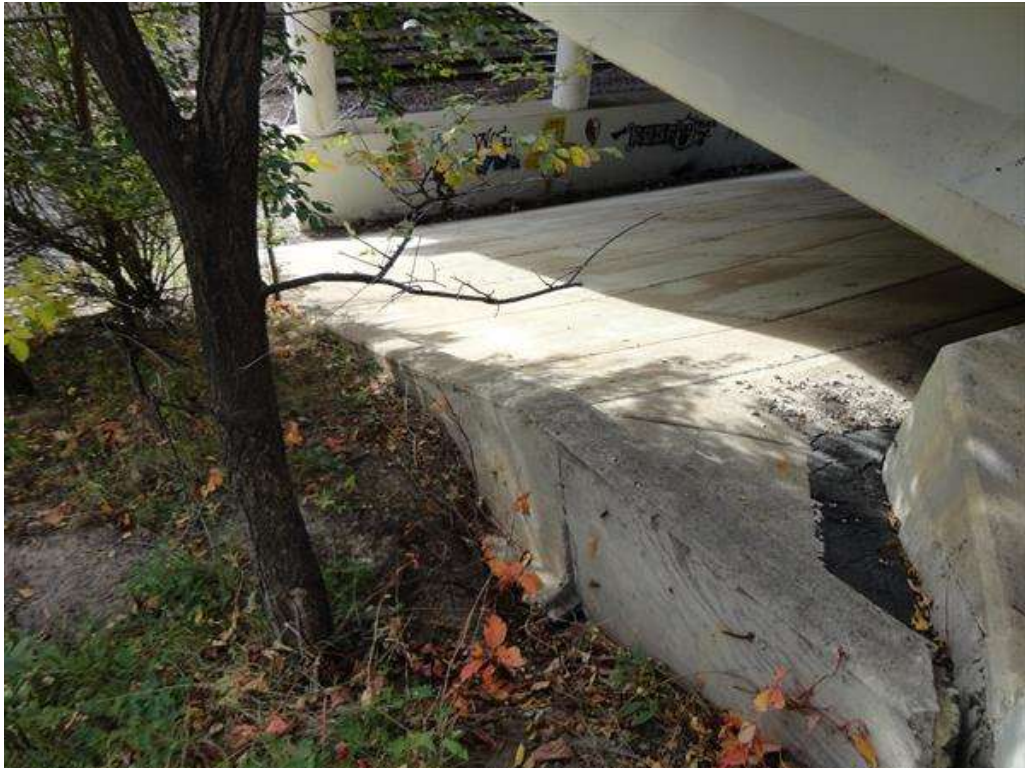
Photo 18 - SW WW slope paving.
