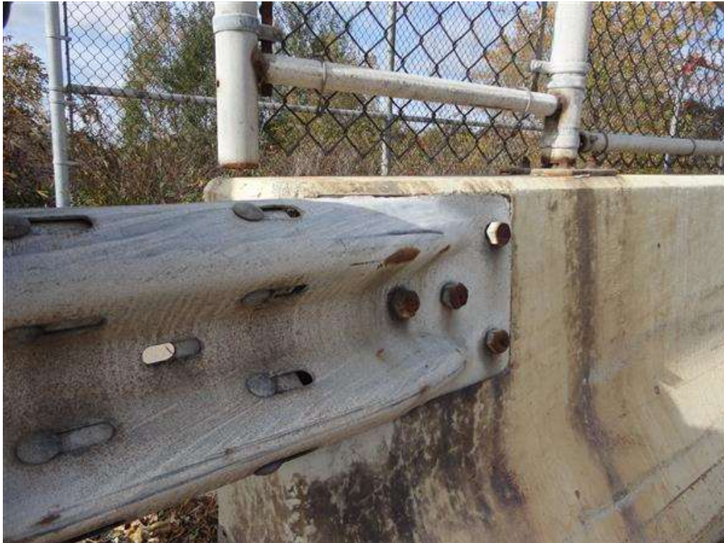
Photo 16 - SW guardrail connection
