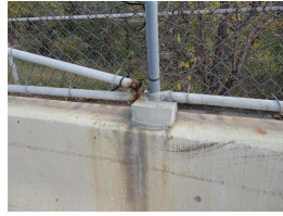
2. East rail repair.JPG
