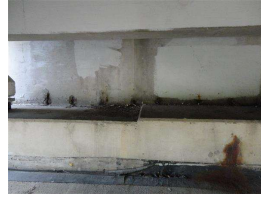
8. South abutment 2.JPG
