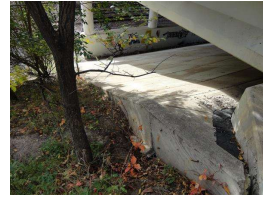
14. SW WW slope paving.JPG
