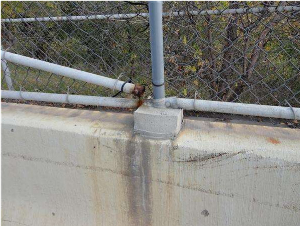
Photo 4 - East rail repair
