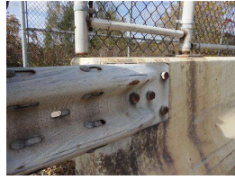
12. SW guardrail connection.JPG
