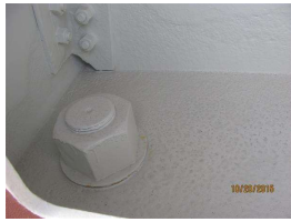
21. 006 Pier 2 Interior at North End New Paint.jpg
