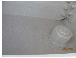
22. 007 Pier 2 Interior at North End New Paint.jpg
