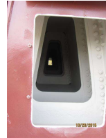
18. 005 Pier 2 Interior at North End New Paint.jpg
