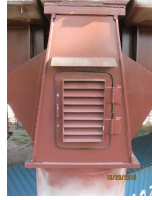
7. 028 Pier 1 South Access Door.jpg
