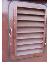
17. 004 Pier 2 North Door.jpg
