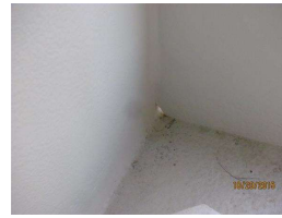
19. 014 Minor Corrosion in the End Diaphragm Corners at the South End.jpg
