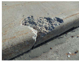
28. N Sidewalk near E end.JPG
