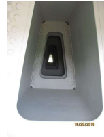
23. 009 Pier 2 Interior at North End New Paint.jpg
