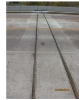
5. 030 Pier 2 Joint Looking South.jpg
