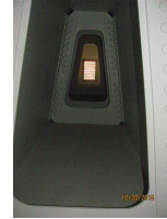
14. 024 Pier 1 Cap Near the North End.jpg
