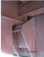
16. 002 Beam 4 Connection to Pier 2 Repainted.jpg
