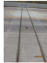
4. 029 Pier 1 Joint Looking South.jpg
