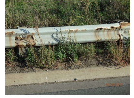
15. northeast approach guard rail.JPG
