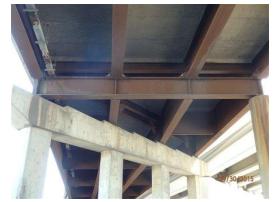
35. steel pier cap 3rd pier.JPG
