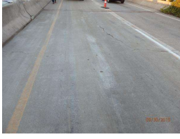
6. approach panels over east end.JPG
