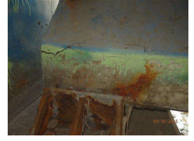
10. east end pre-stressed beam.JPG
