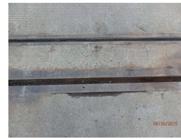
39. upper deck east abut section 12.JPG
