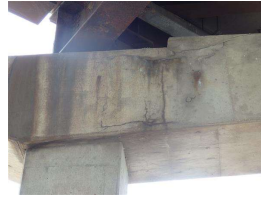
48. 4th Pier cap from the W.JPG
