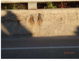
11. jersey barrier 300ft c.s. #2.JPG
