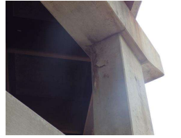
53. Column, 6th pier from the W.JPG
