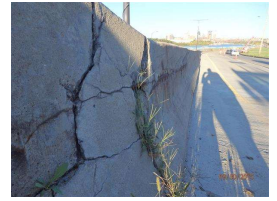
30. southwest approach jersey barrier.JPG
