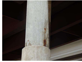
52. Column, 4th pier from the W.JPG
