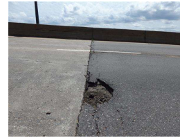
59. Roadway at W approach.JPG
