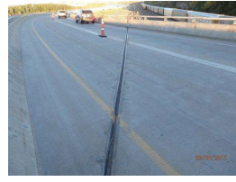
19. section #5 strip seal.JPG
