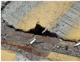
11. second hole in deck south abut..JPG
