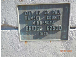
1. bridge ID plate.jpg
