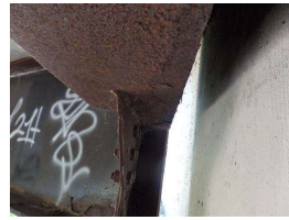
14. south abut. east end bottom of diaphragm flaking rust.JPG
