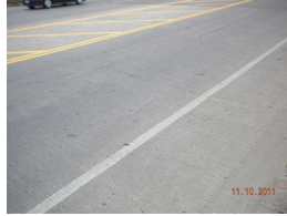
8. approach panel W.end_1.jpg
