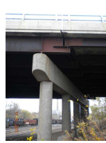
68. joint - pier 1_2.jpg
