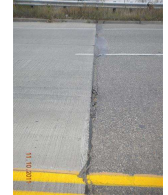
10. approach panel W.end_3.jpg
