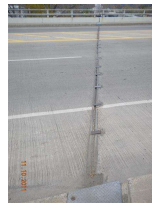
67. joint - pier 1_1.jpg
