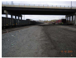
2. 2011 elevation view center_span.jpg
