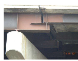
69. joint - pier 1_3.jpg
