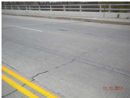
11. approach panel W.end_4.jpg
