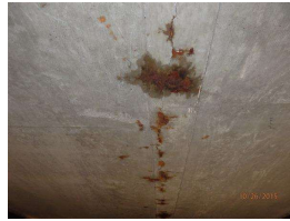
7. 020 W end underside of deck, center span..JPG
