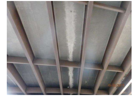
10. 022 W end underside of deck center span..JPG
