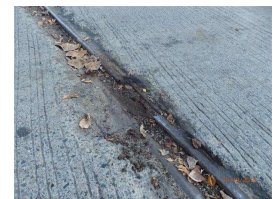
25. Joint at W end (1)..JPG
