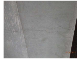
9. 021 W end underside of deck..JPG
