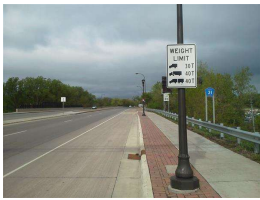
1. 009 Load Posting Sign 62526 WB_Maryland - relocated.jpg
