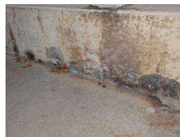
23. Concrete rail, W end..JPG
