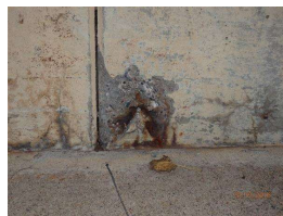
22. Concrete rail, midspan..JPG
