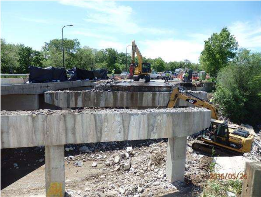
Photo 2 - 2016 bridge Re-hab. Project.jpg
