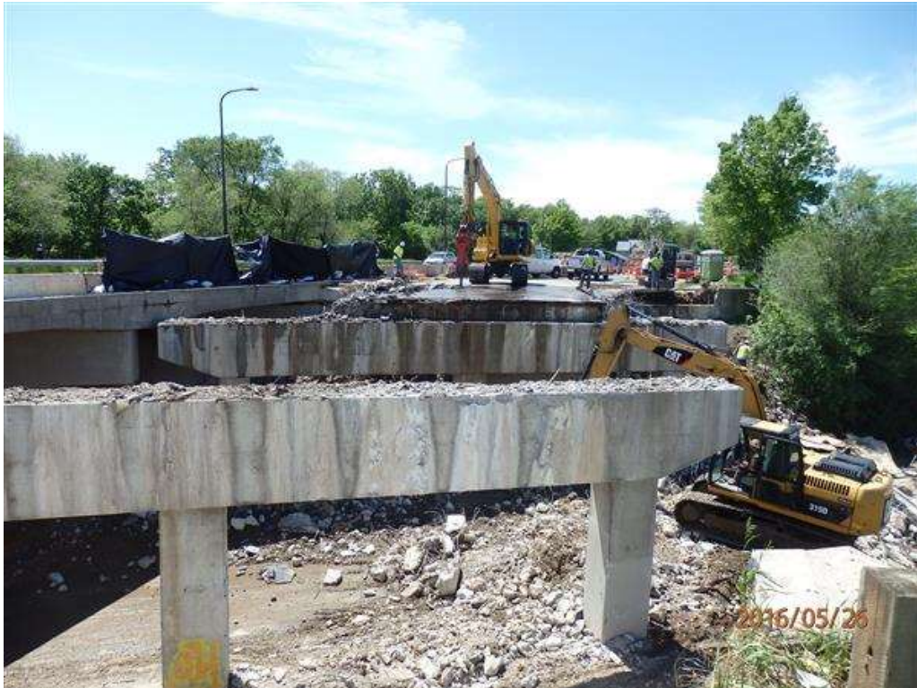
Photo 2 - 2016 bridge Re-hab. Project.jpg
