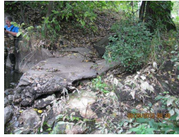
3. East end spillway.JPG
