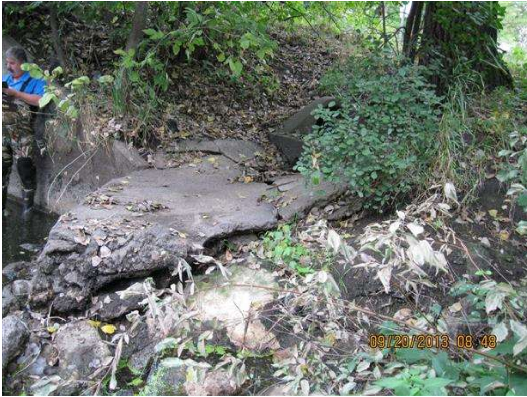
Photo 3 - East end spillway 2013
