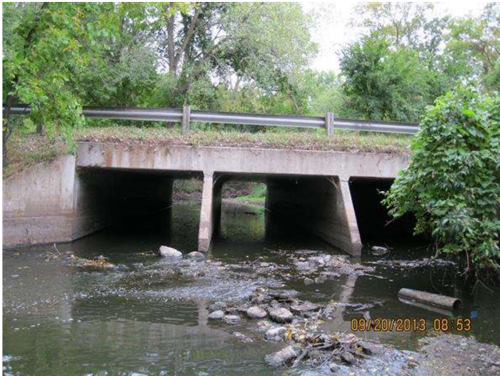
Photo 6 - west end culverts 2013
