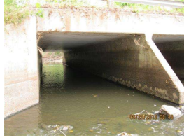
7. west end north culvert.JPG
