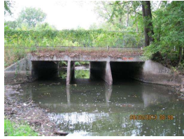
2. east end culverts.JPG
