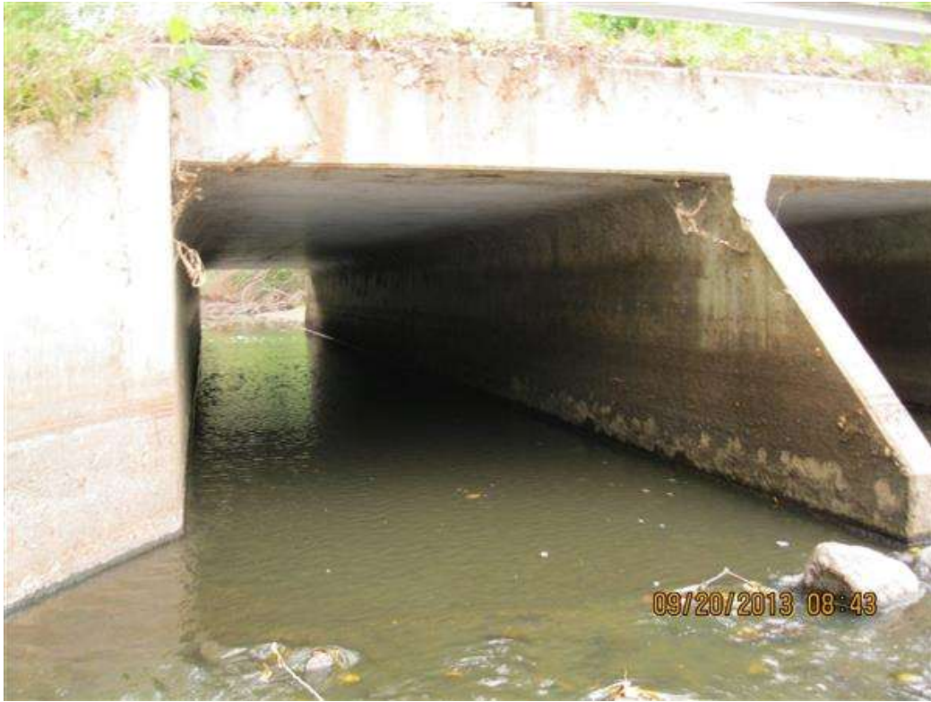
Photo 7 - west end north culvert 2013
