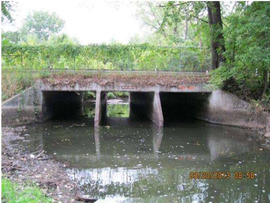
Photo 2 - east end culverts 2013
