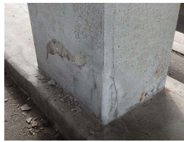
3. Center pier assy, 2nd column from E, N side.JPG
