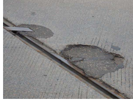
7. NB lane at S expansion joint.JPG
