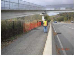
6. CB repair area_1.jpg
