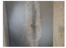
20. Under W sidewalk near the N end.JPG
