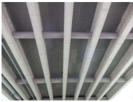
21. Underdeck, mid span facing S.JPG
