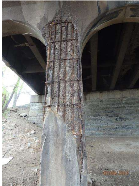
Photo 14 - pier 2 - column W.side
