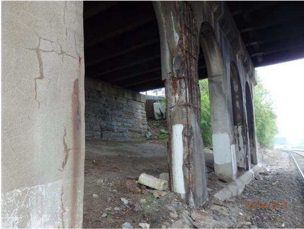
Photo 15 - pier 2 - columns East view
