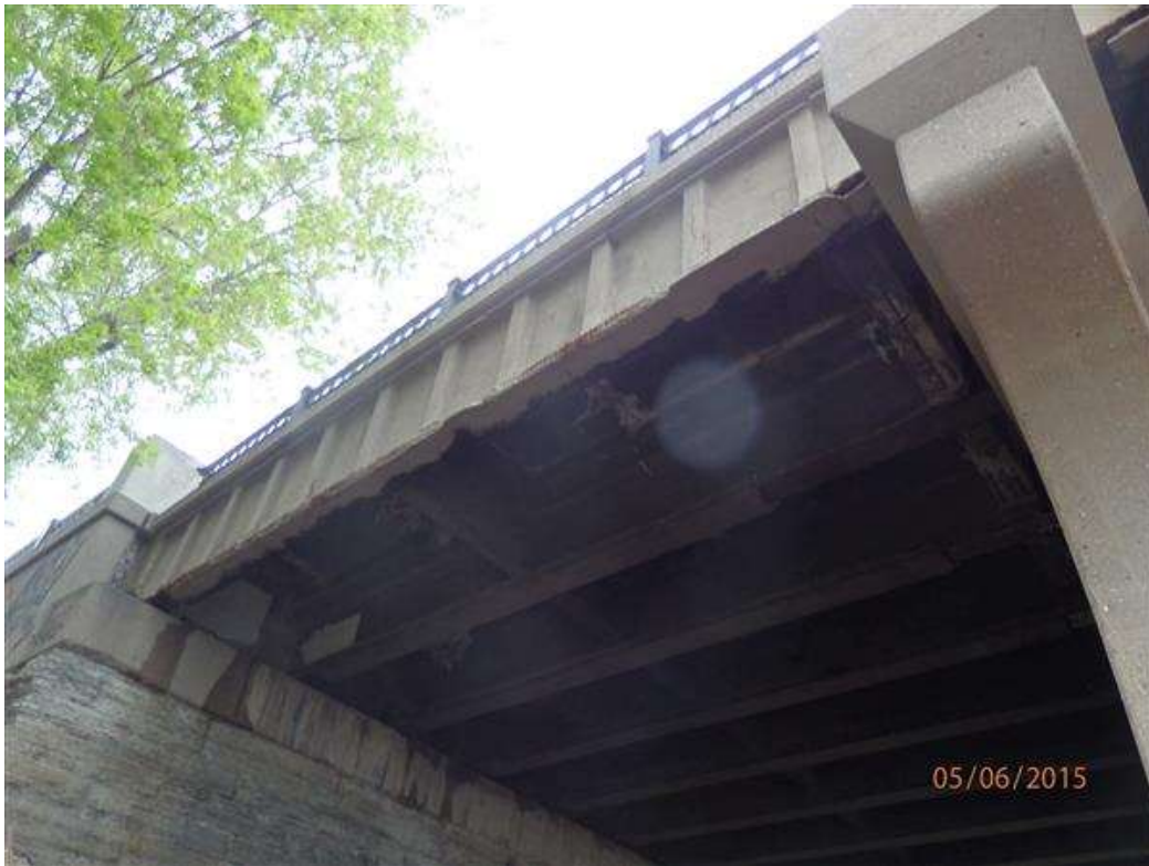
Photo 5 - abut beam - NW.end
