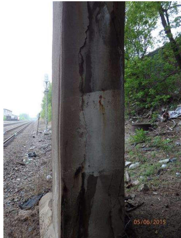
Photo 12 - pier 2 - column E.side
