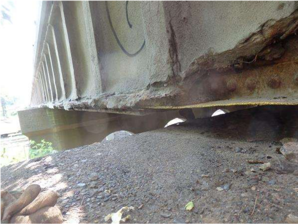
Photo 7 - abut NE fascia beam
