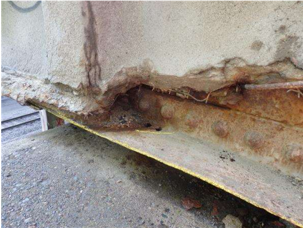
Photo 8 - abut NE fascia beam (2)
