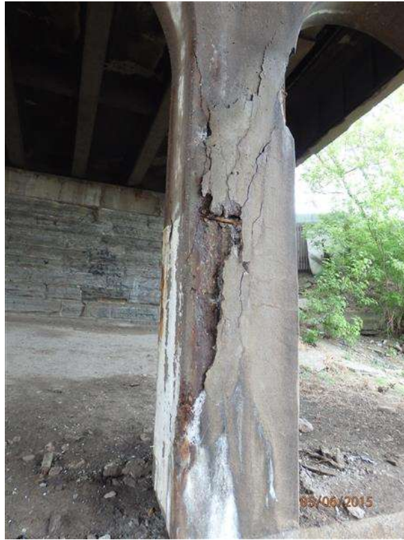
Photo 13 - pier 2 - column W.inner.side
