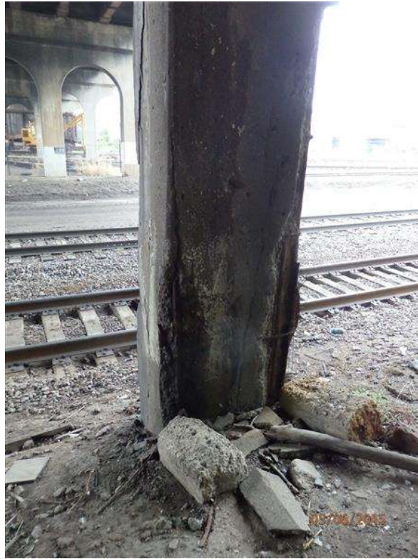
Photo 11 - pier 2 - column E.inner.side
