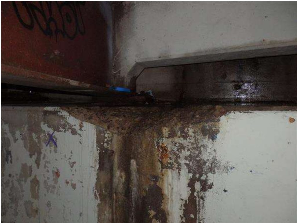
Photo 28 - S Abutment, W end
