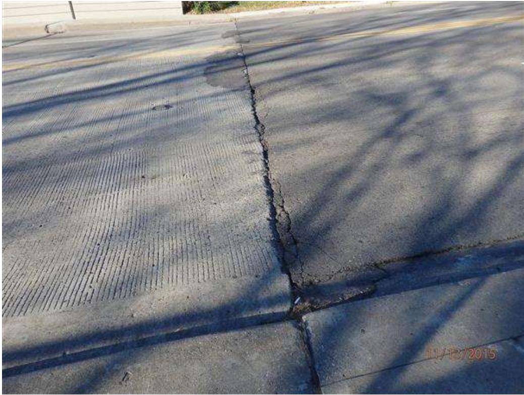
Photo 11 - liquid poured joint north approach
