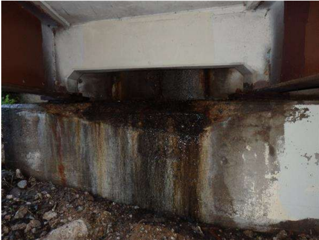
Photo 26 - S Abutment, E end (1)
