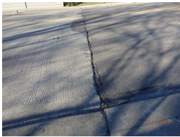
11. liquid poured joint north approach.JPG
