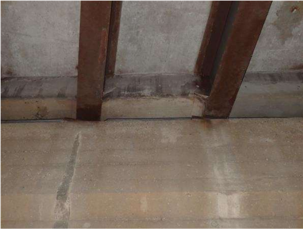
Photo 23 - Diaphragm at pier 4 (1)
