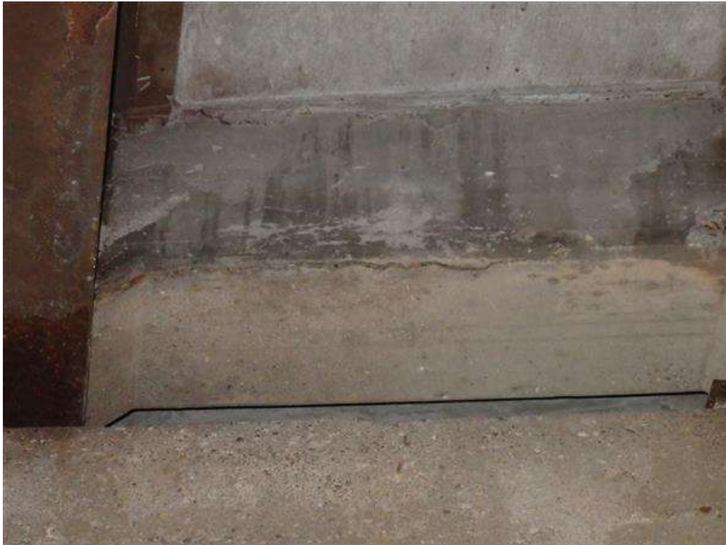
Photo 24 - Diaphragm at pier 4 (2)
