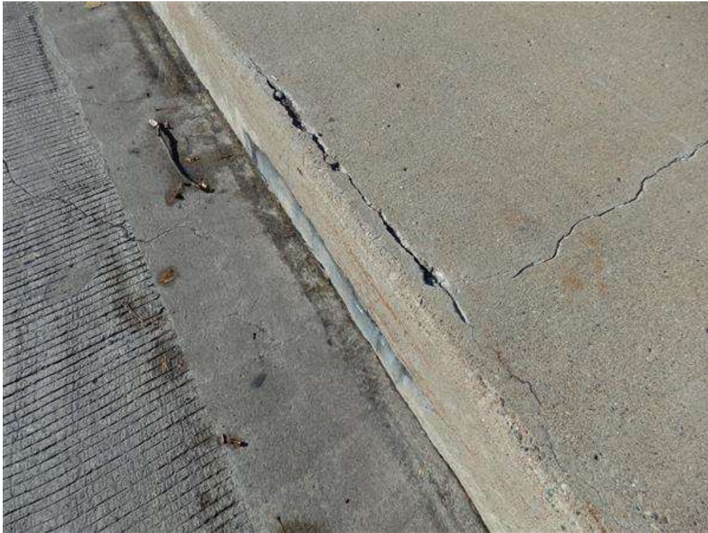
Photo 30 - Southbound curb at S end
