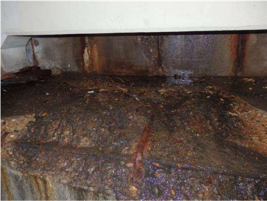
Photo 27 - S Abutment, E end (2)
