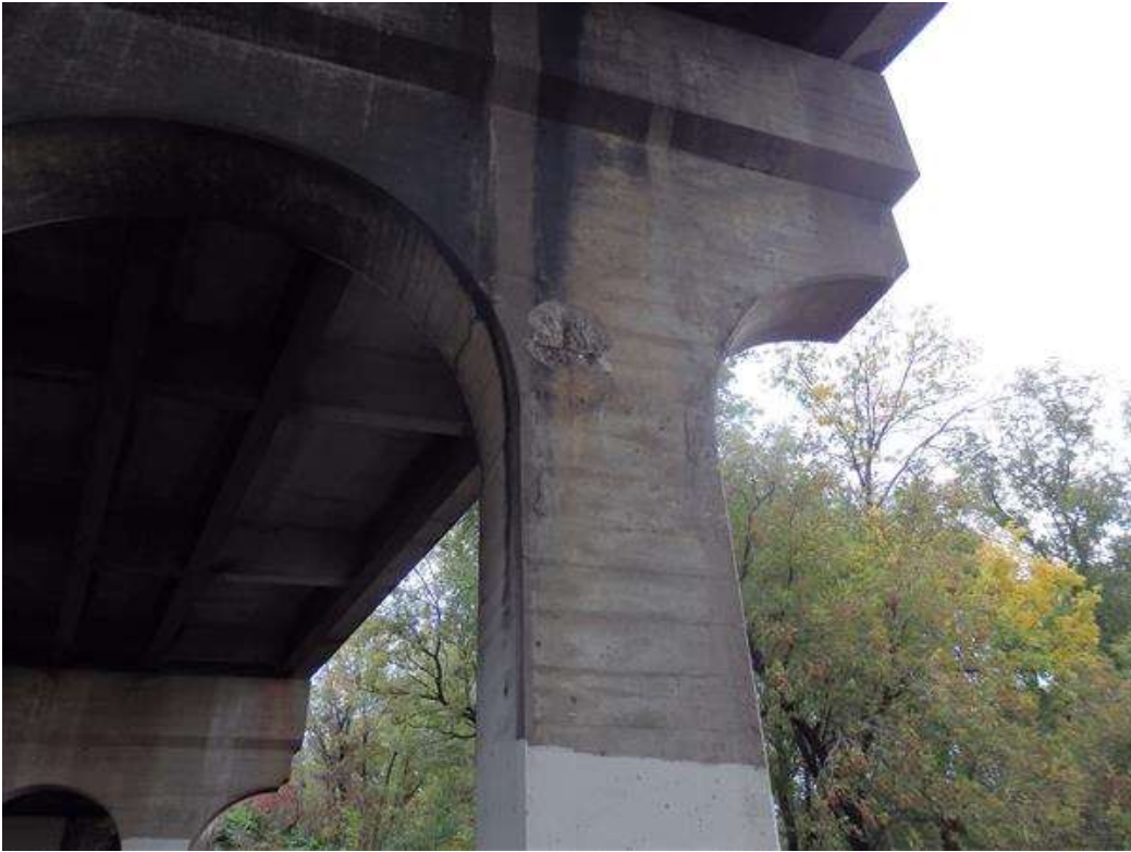
Photo 25 - Pier 3, S face
