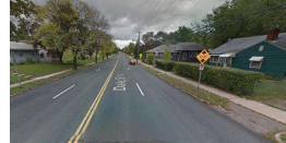
24. NB pre-warning signage.PNG
