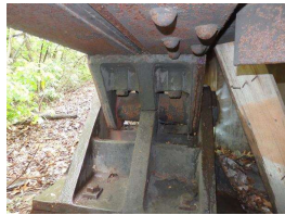
12. south west bearing west abutment.JPG
