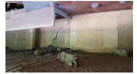
5. E concrete abut back wall.jpg
