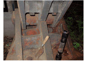
10. north west bearing west abut.JPG
