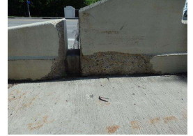
10. Concrete rail, SW end, sidewalk side.JPG
