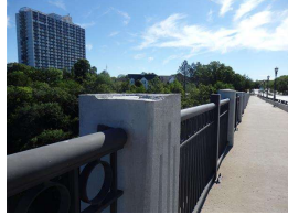
7. Concrete rail (1).JPG
