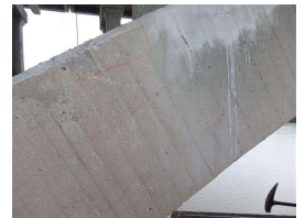
25. Span 9-10, Facing N, below spandrel O.JPG
