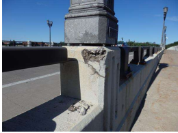
6. 8th light standard from the E, N side of bridge.JPG
