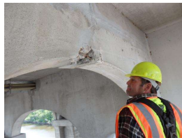
22. Span 8-9, Facing N, Between spandrel A-B.JPG
