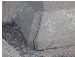
23. Span 8-9, Facing N, Spandrel C.JPG
