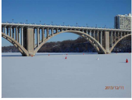
36. Elevation view - Center River Span.JPG
