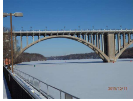
38. Elevation view - W. River Span.JPG
