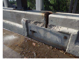
9. Concrete rail, SW end, drive lane.JPG
