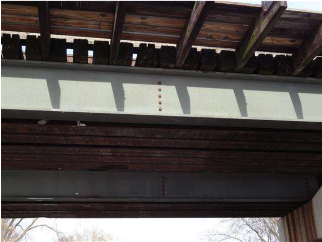
Photo 8 - 2937 NB girders from south 2012
