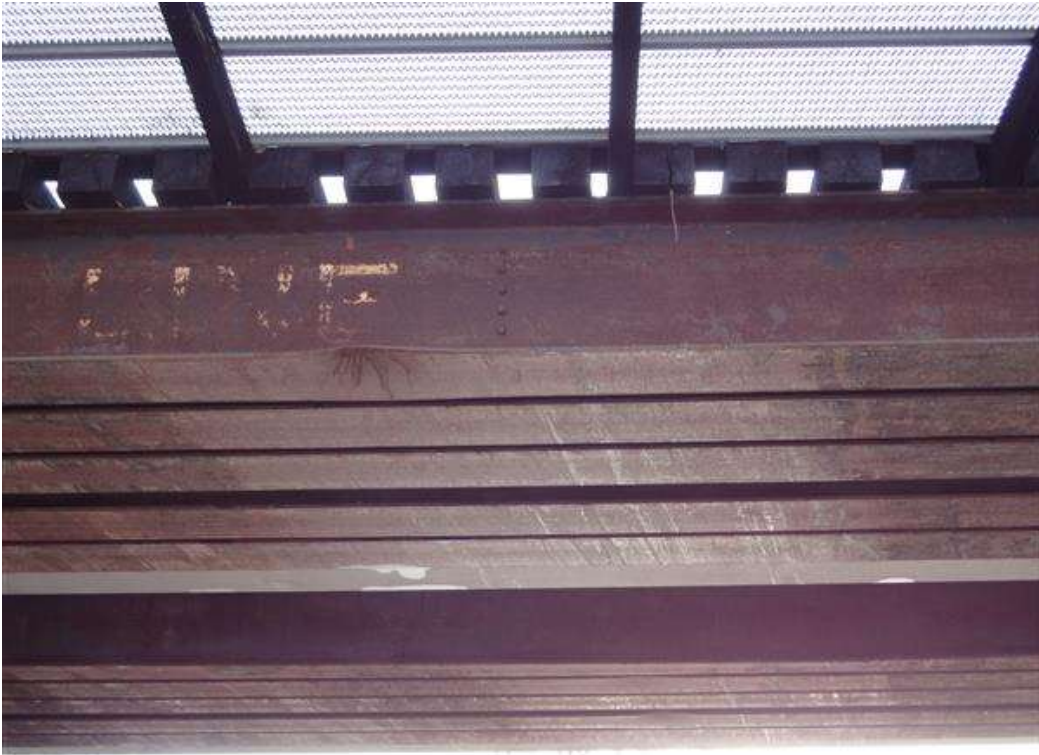
Photo 6 - 2937 girders from north 2012
