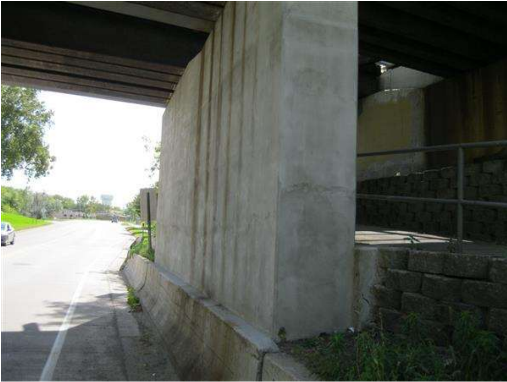
Photo 26 - west pier wall 2014
