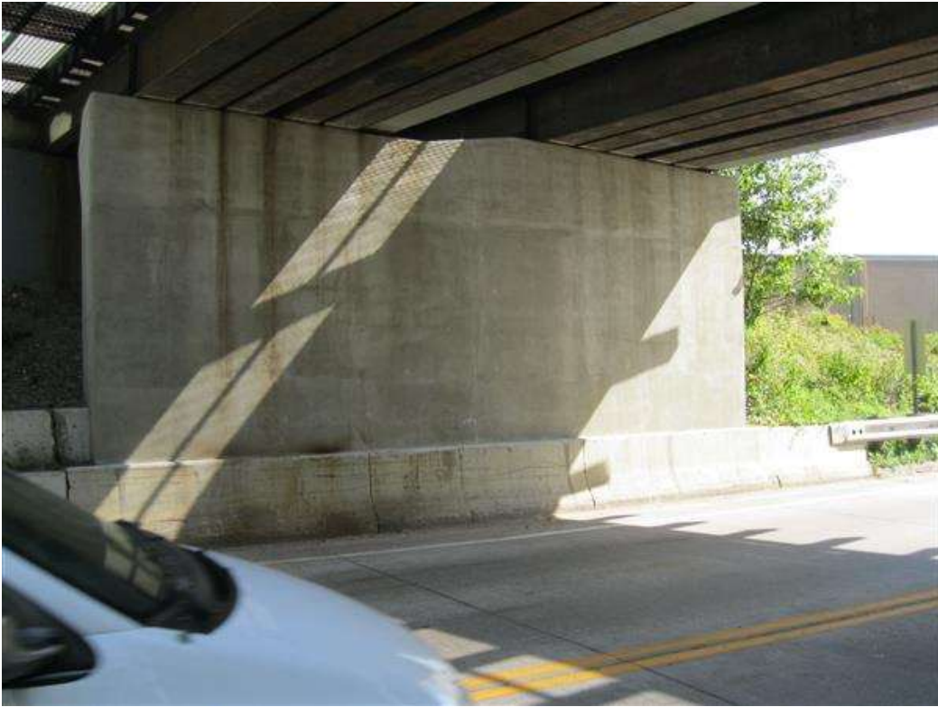
Photo 22 - east pier wall 2014
