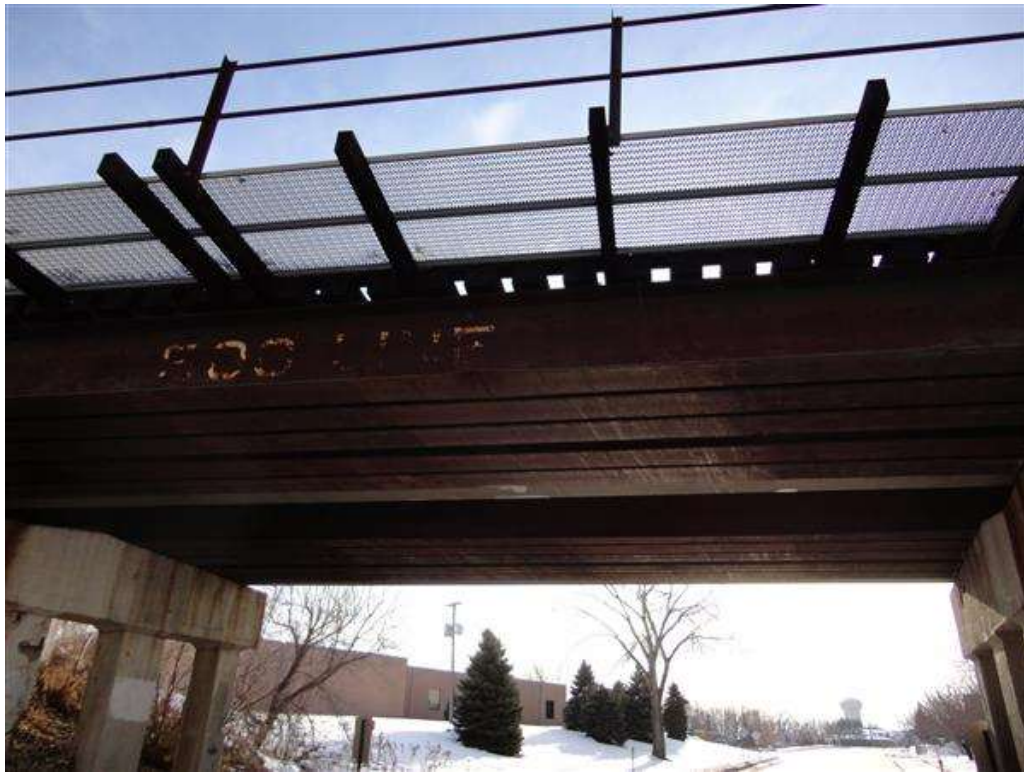
Photo 9 - 2937 SB girders from north 2012
