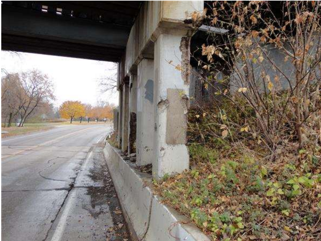
Photo 2 - 2937 E Pier Culumns 2012
